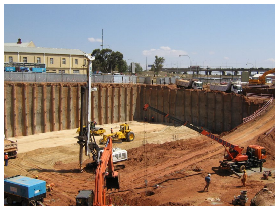
Images showing the construction of building in 2007.
