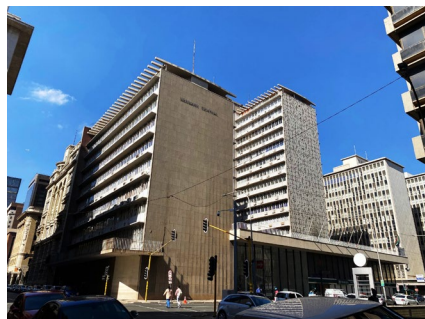
VIEW OF THE NORTH WEST CORNER OF THE BUILDING
