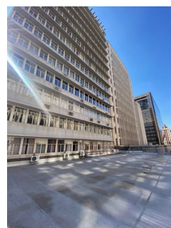
VIEW FROM ROOF AREA ON MAIN STREET
